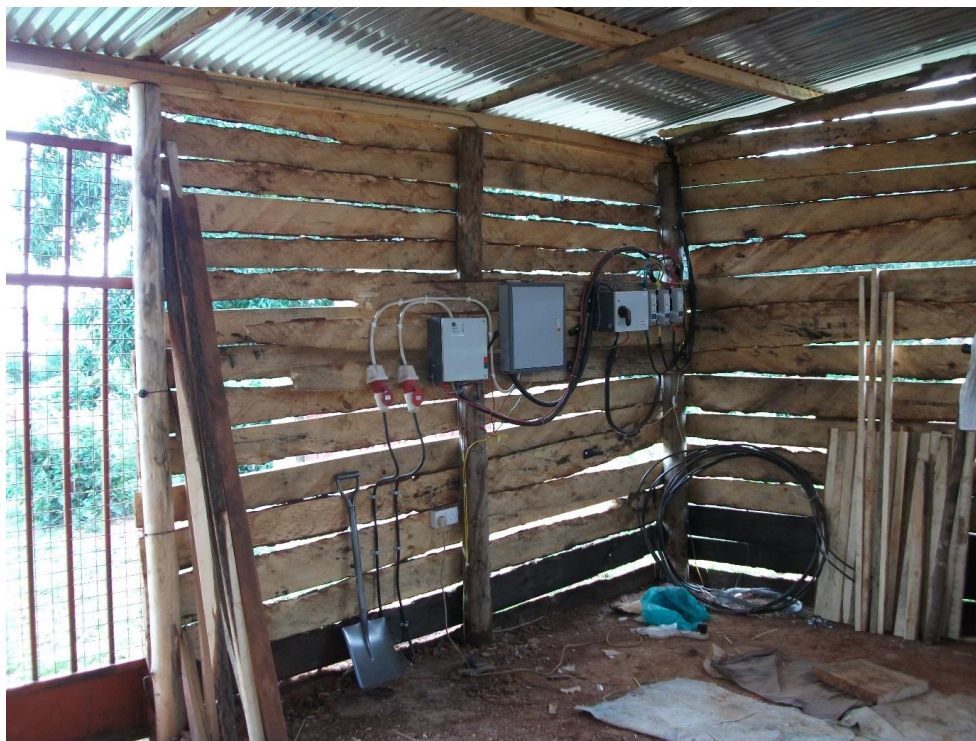
Electrical wiring in the workshop and it is three phase electricity for industrial work.
