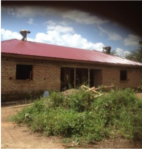
Roofing at resource center
